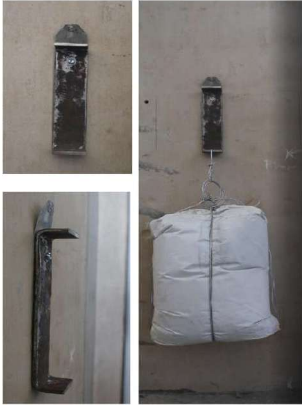
Fig 22. Pull down test
