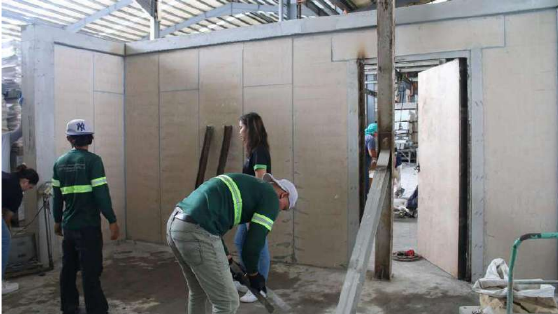
Fig 1. Litepanel™ wall specimen for performance test
